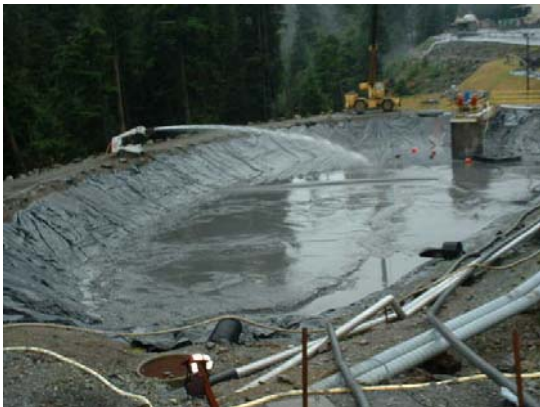
Eagle has the capability to pump difficult materials in remote locations.
