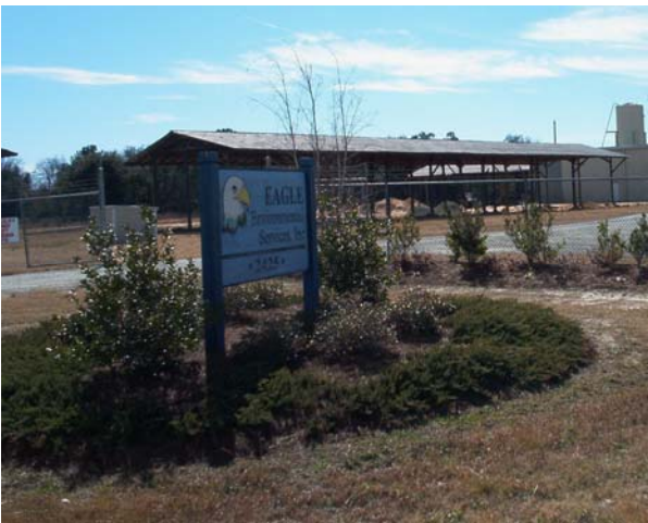
Eagle's fully permitted waste processing and recycling facility located in
