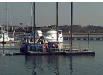
Eagle provides sediment removal at a private marina.
