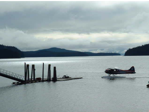
Eagle recently completed a dredging project in Alaska for Kennecott that was in a remote location only accessible by boat or float plane.
