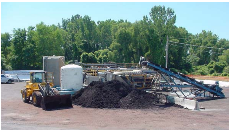
Multiple press location featuring six 2.0 Meter Belt Press Dewatering Skids and auxiliary equipment.
