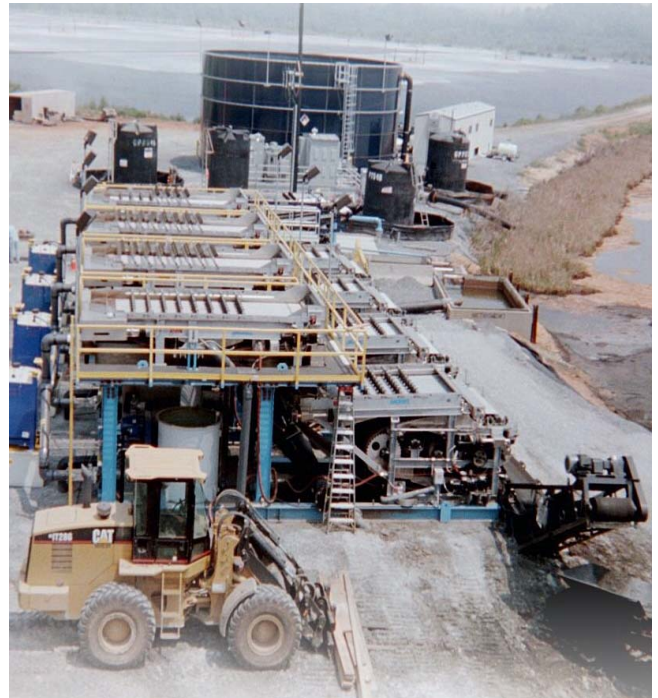
Eagle designed, constructed, and operates a sludge dewatering facility at a pulp and paper mill in the Southeast. This plant operates continuously 24 hours per day; 365 days per year, and has the capacity to continually dewater five million gallons of sludge daily.
